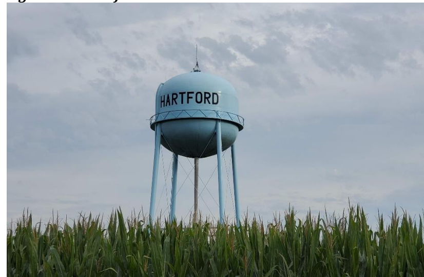
Figure 6-5: Hartford Water Tower
