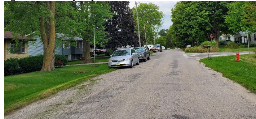
Figure 6-2: Example of Seal Coat Street
