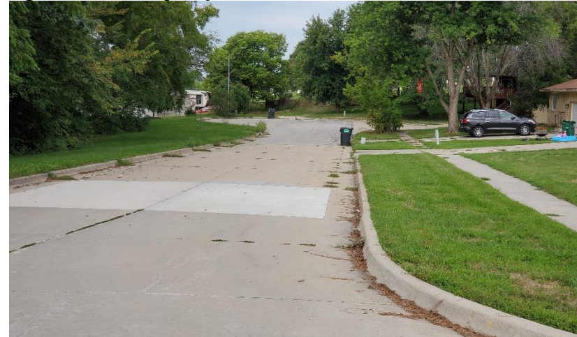
Figure 6-1: Example of Concrete Street with Curb + Gutter
